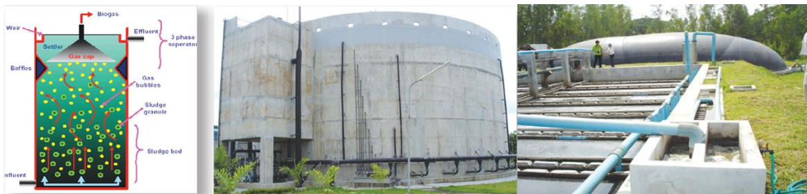
Figure 5 UASB and H-UASB system
