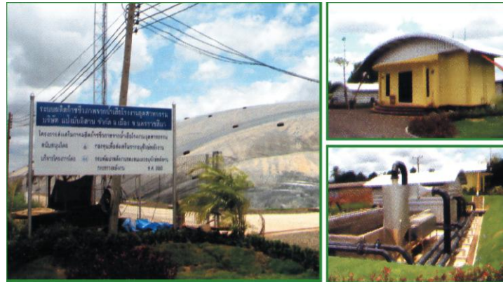
Figure 6 I-san Tapioca Flour Ltd.'s biogas production and water treatment systems
