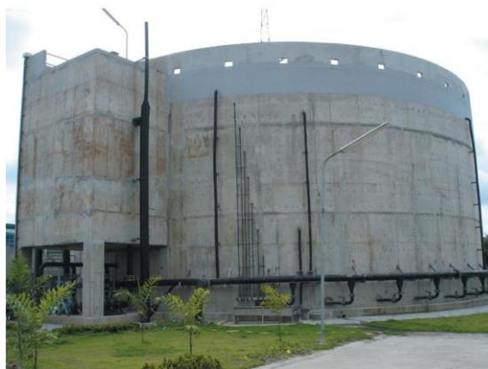
Figure 1 Up-Flow Anaerobic Sludge Blanket (UASB) system
