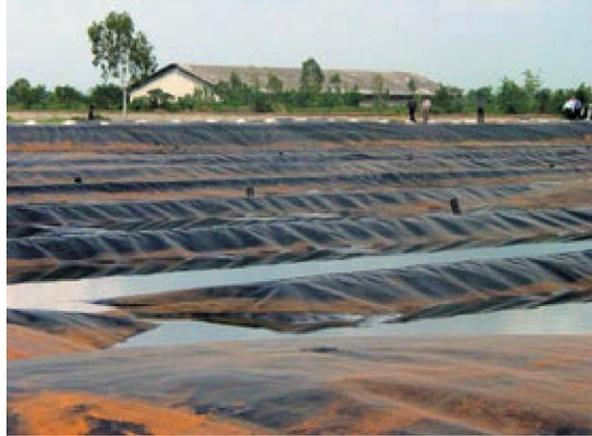
Figure 4 Anaerobic Baffle Reactor (ABR) system
